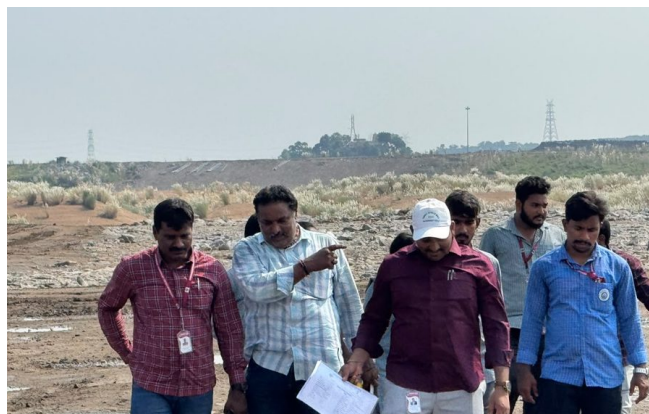
Photo 8. Walking through the head works area during the site visit
