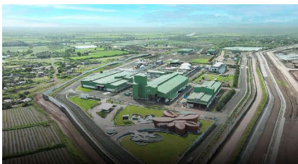
Aerial view of Reliance Bioenergy Plant
